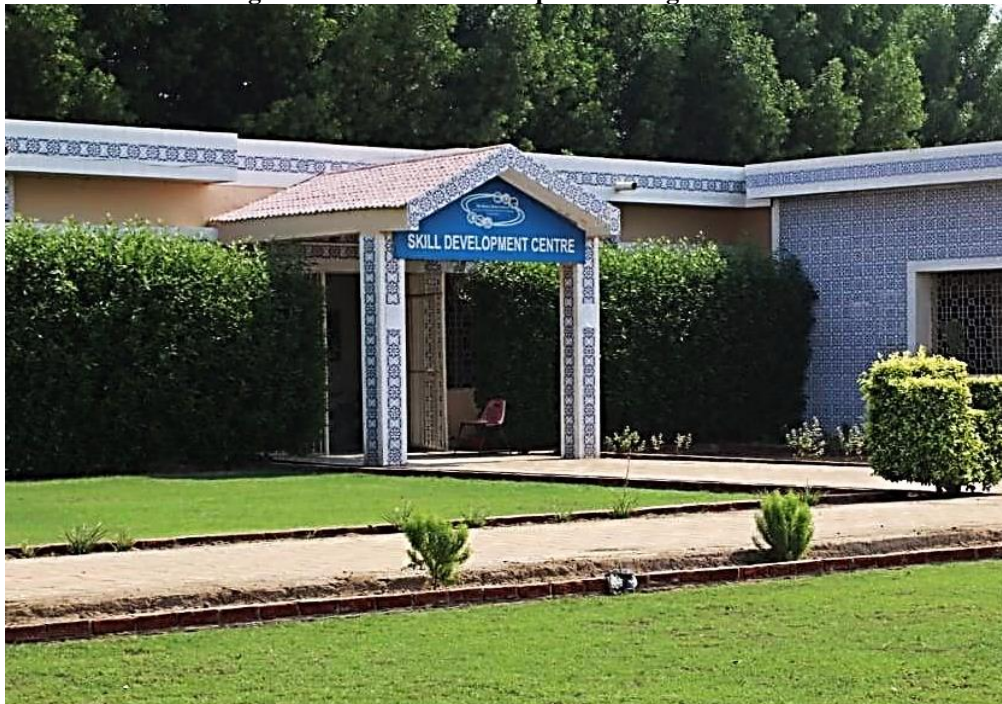
Existing Structure of Main Campus Buildings at BBSUTSD
